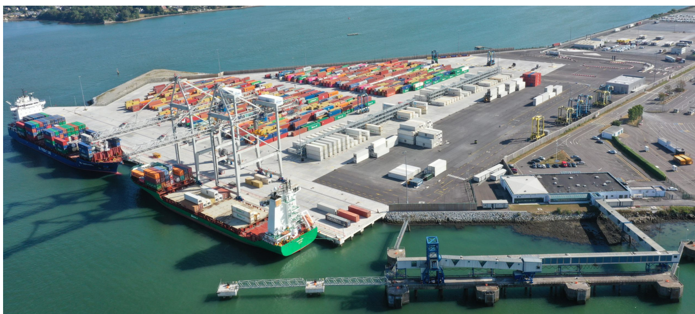
Figure 2: Port of Cork Expansion, Ringaskiddy (Credit: Port of Cork)
