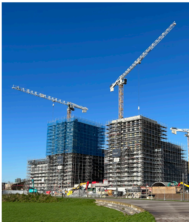
Figure 3: Housing Delivery in Cork Docklands
