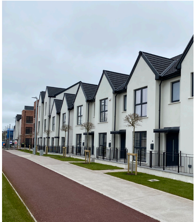
Figure 8: New Residential Development
