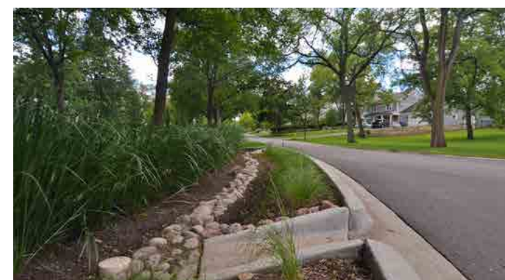
SuDs features - including swales, ditches and bioretention features
